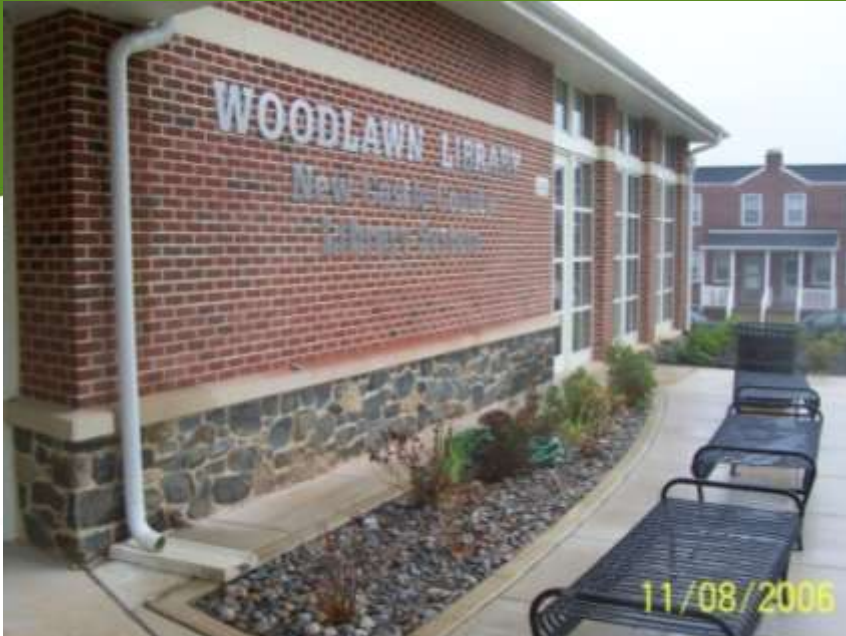
Rainwater flows off the rooftop and into the downspout...
